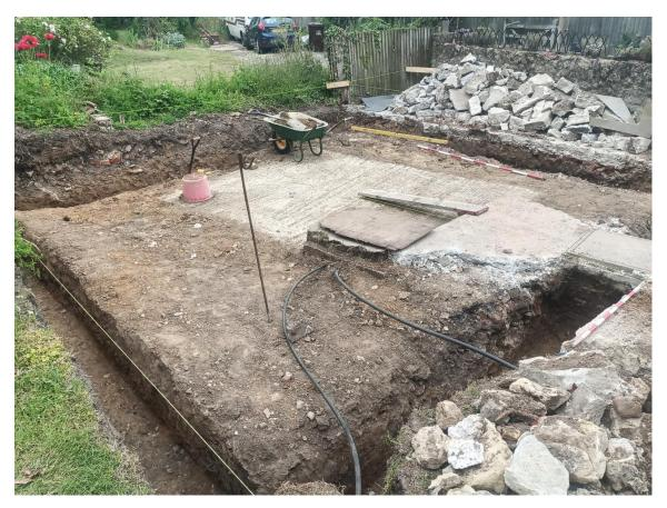
Plate 3. Foundation footing (looking SSW)
